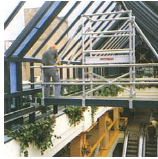
Walkways can be mounted on rollers to provide mobile Access Gantries.
